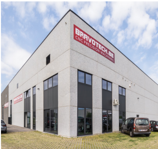
In 2015, Bram Vergote purchased the first workshop of a three-building complex in Oudenaarde.
